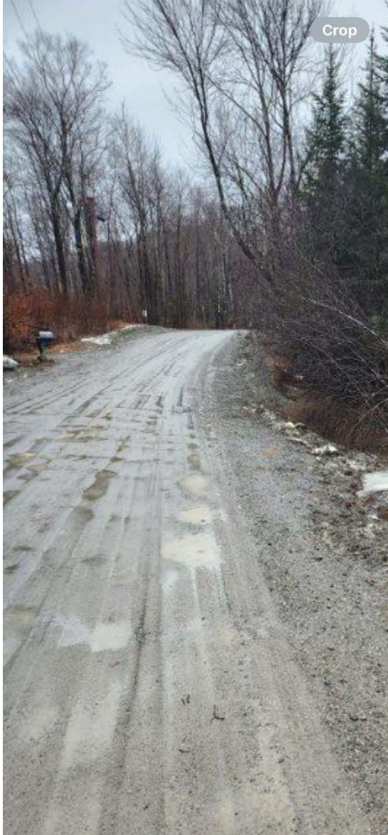
Segment 142057 Looking North
